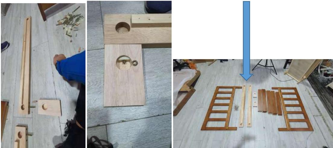
Then, join 2 bars and the leg, which is the front frame of the sofa, please check the arrow to find the parts.
